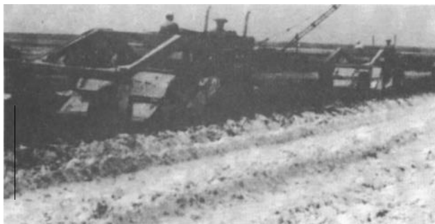
Figure 4-38. Train of rotary mixers.
