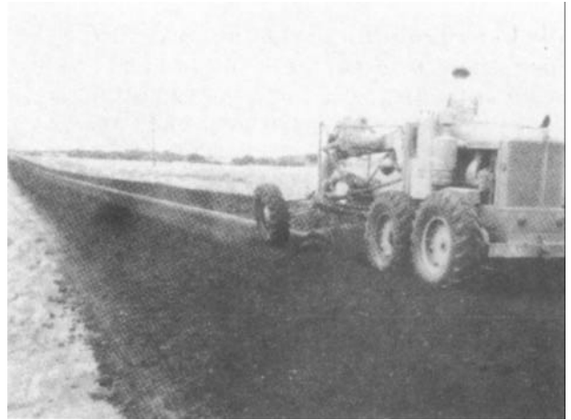
Figure 4-50. Mixing with motor grader.
