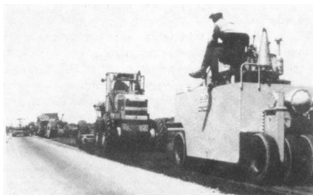
Figure 4-52. Spreading and compacting train.
