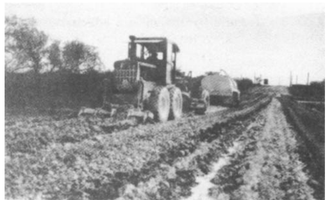
Figure 4-33. Grader-scarifier cutting slurry into stone base.
