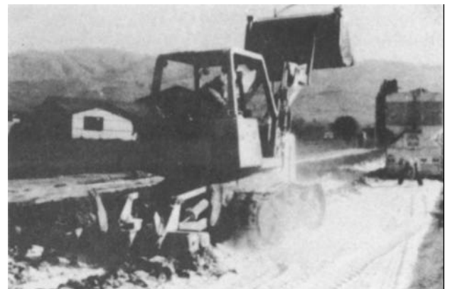
Figure 4-19. Scarifying existing clay subgrade with lime on city street project.
