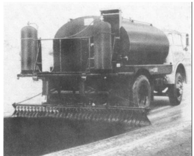
Figure 4-51. Distributor applying asphalt.
