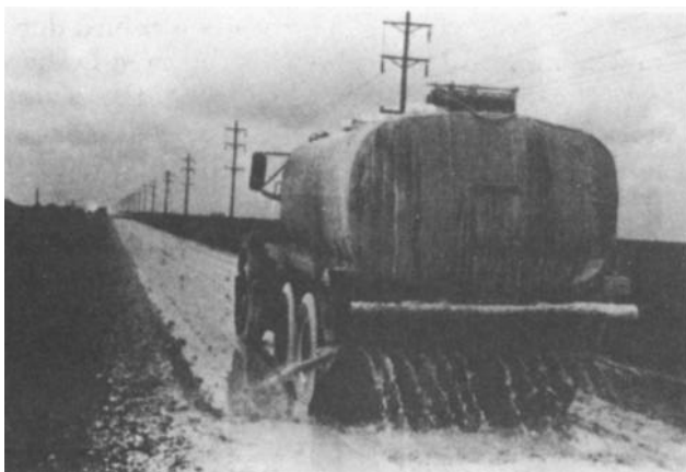
Figure 4-31. Spreading of lime slurry.
