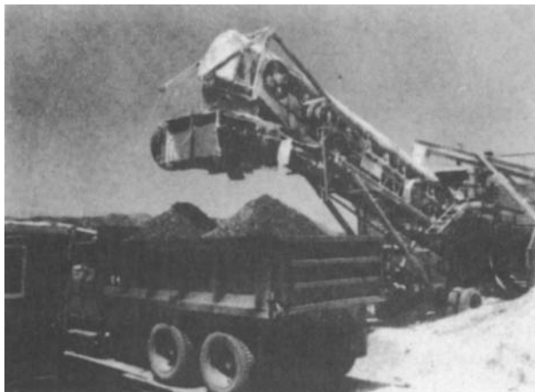
Figure 4-20. Lime-treated gravel with lime fed by screw conveyor.
