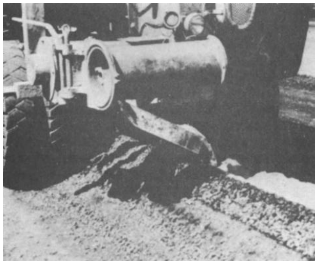
Figure 4-9. Windrow-type mechanical spreader placing cement on windrow.
