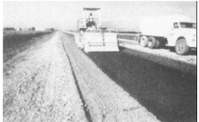
Figure 4-39. Rotary mixer on primary road project.
