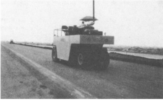
Figure 4-42. Pneumatic roller completes compaction of LCF base.
