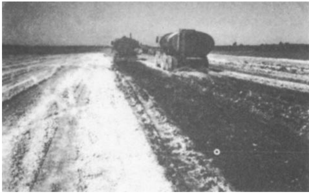
Figure 4-35. Watering of lime-treated clay on airport project.
