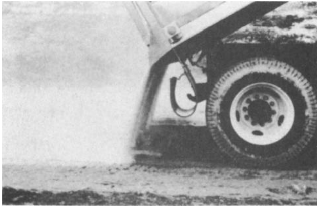
Figure 4-28. Spreading of granular quicklime.
